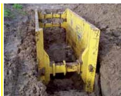
PANEL  $t_{PL} = 127\text{mm}$
